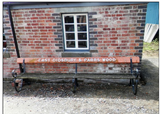
The dilapidated bench outside the weighbridge before restoration began
