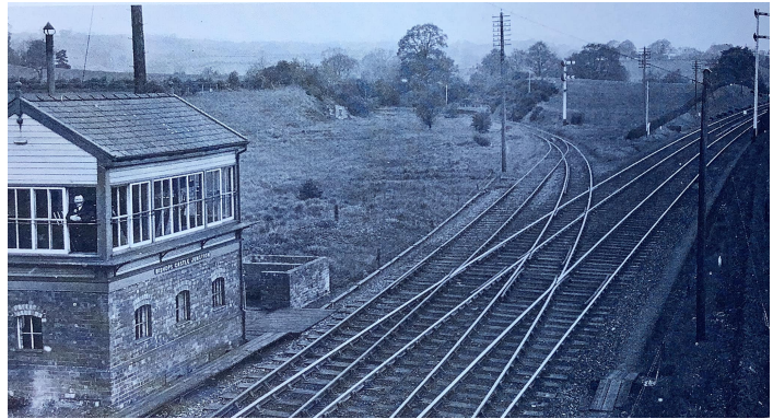
Stretford bridge junction , the halt can be seen centre of the photo to the left of the telegraph pole between the two bushes
