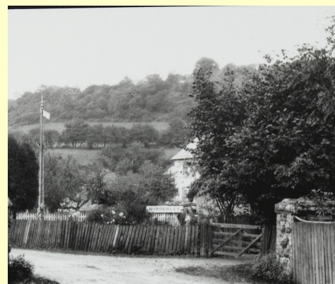
The signal in situ at Horderley station
