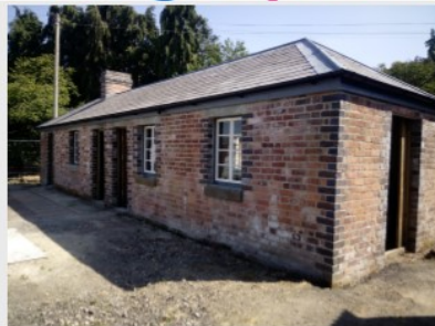
The Railway Weighbridge Building Station Street, Bishop's Castle, SY9 5AQ
