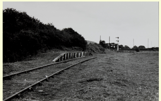
Stretford Bridge Halt at the time of the BCR
