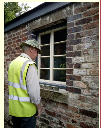
Roger checking that the window is straight before securing
